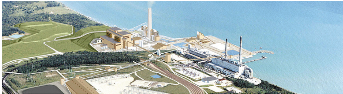
Elm Road Generating Station.
