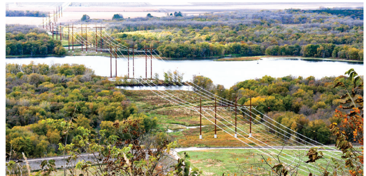
CapX2020’s Hampton-Rochester-La Crosse transmission project crosses the Mississippi River.
