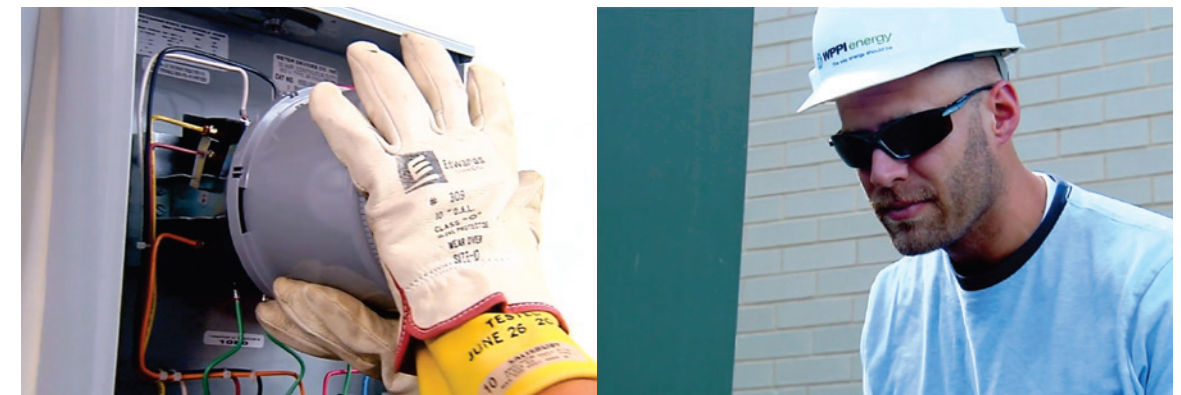
The WPPI shared meter technician service.
