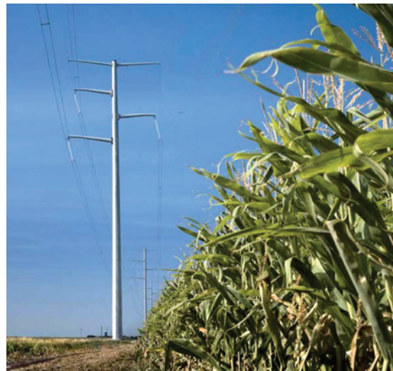
CapX2020 works to strengthen the region's transmission grid.
