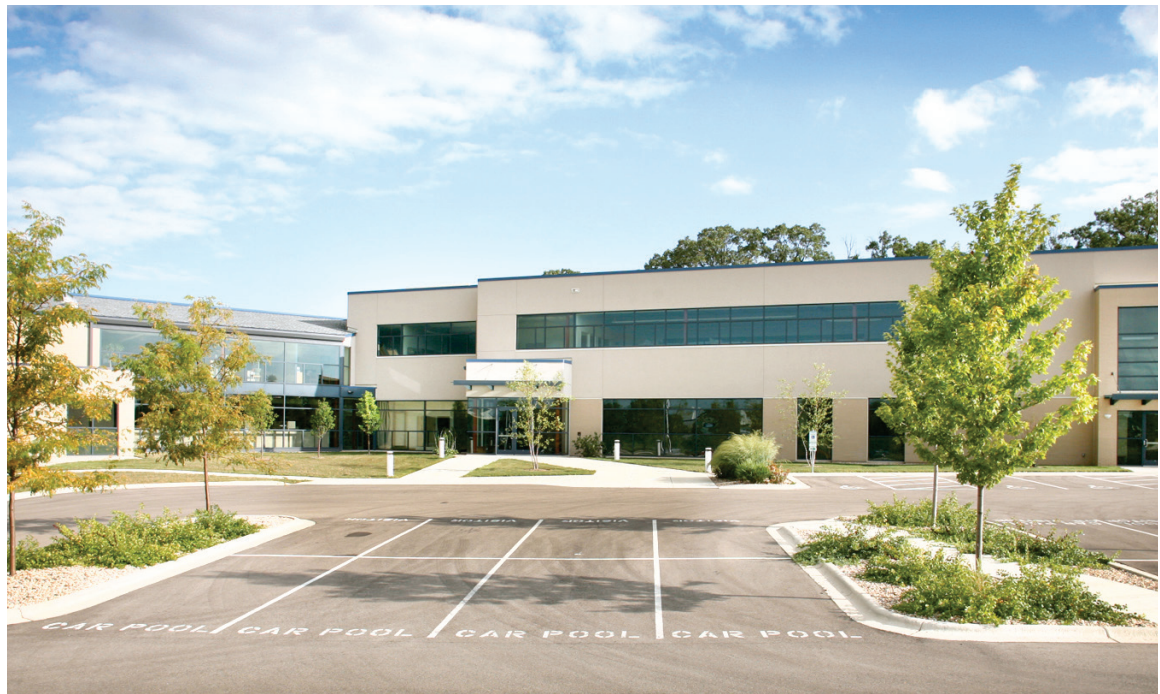
WPPI's LEED "Gold," ENERGY STAR certified office and operations facility is among the most energy efficient buildings in the nation.
