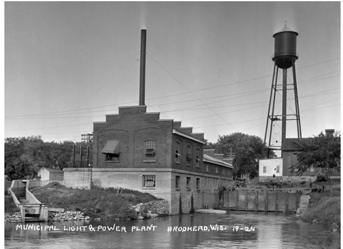
The Municipal Light and Power Plant of Brodhead, Wis., in 1924. Wisconsin Historical Society, WHS84812.
