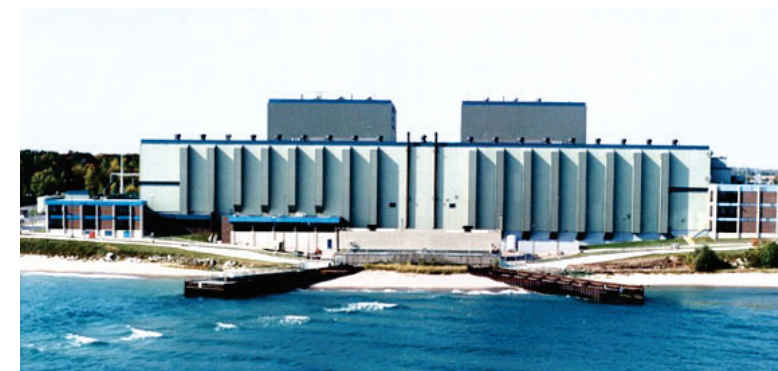
Point Beach Nuclear Power Plant.
