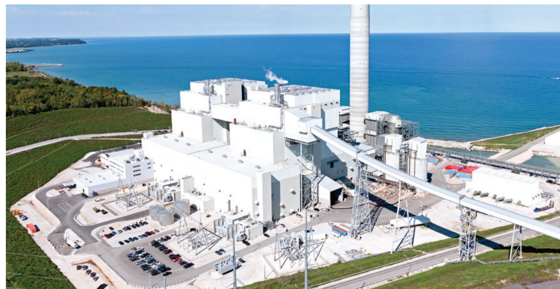
Elm Road Generating Station.
