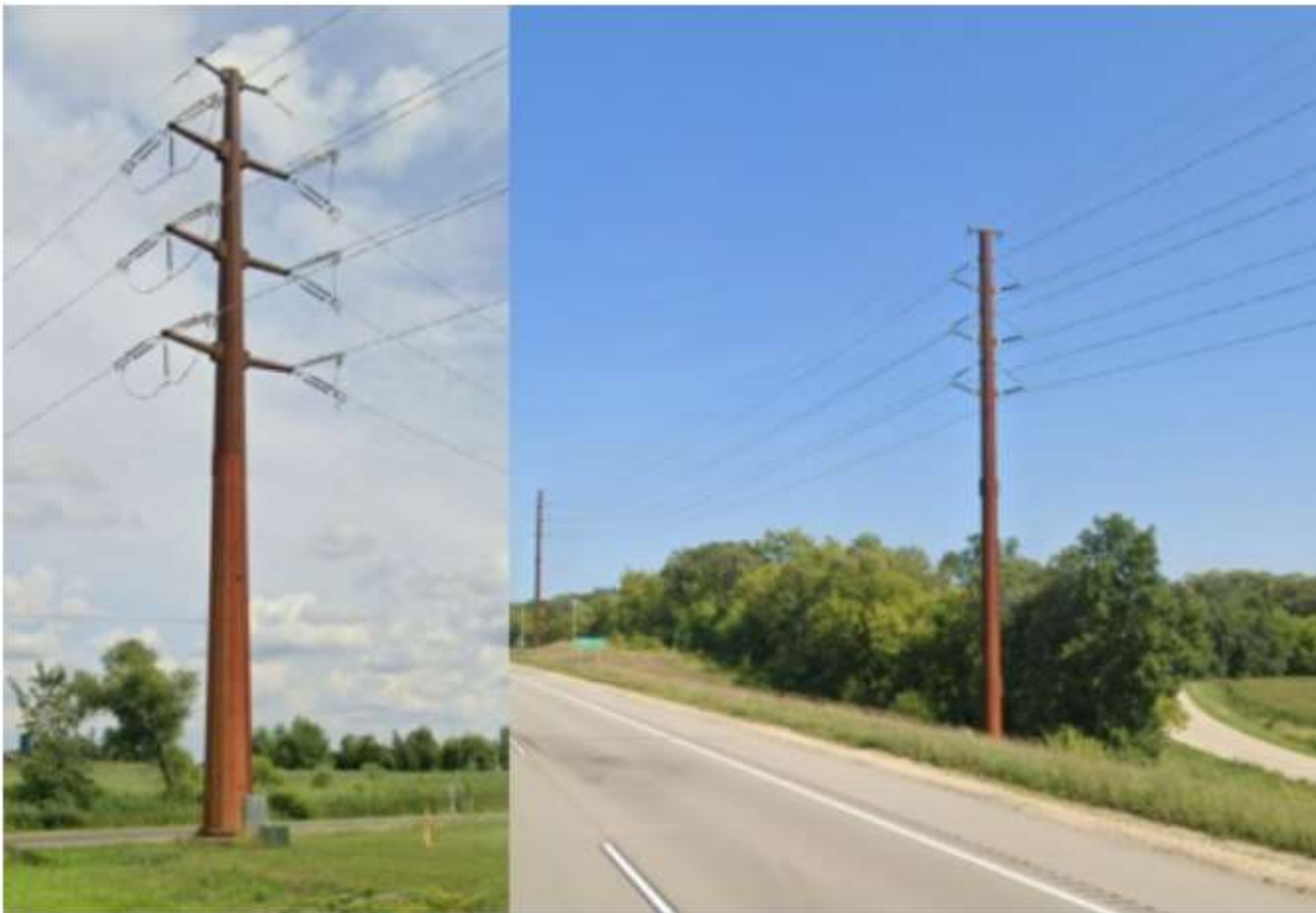
Towers Like These are Proposed by American Transmission Company for the Plymouth Reliability Project. Images Courtesy of ATC
