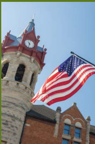
STOUGHTON UTILITIES 6TH (6%)
